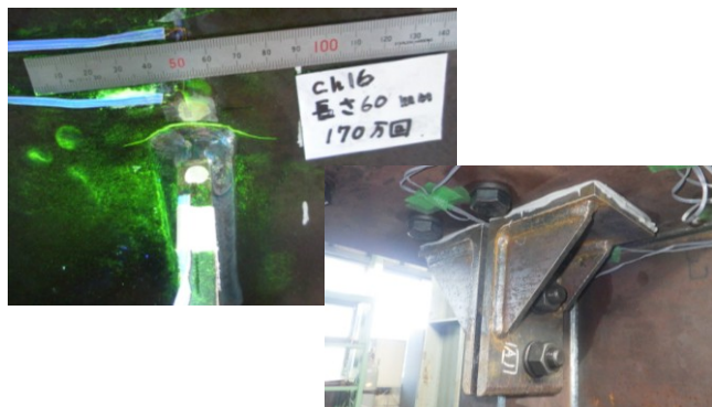
図-6 疲労き裂の一例と補強状況
